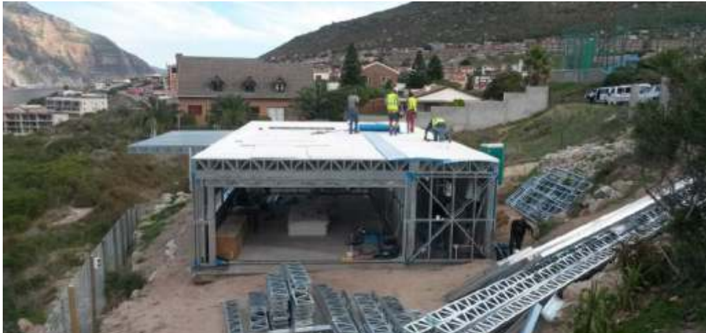
Installation of MGO Boards
