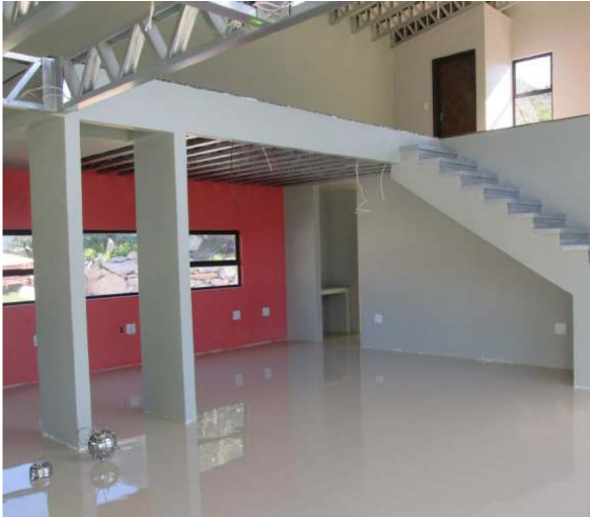
Completed Suspended Light Steel Frame Joist Floor
