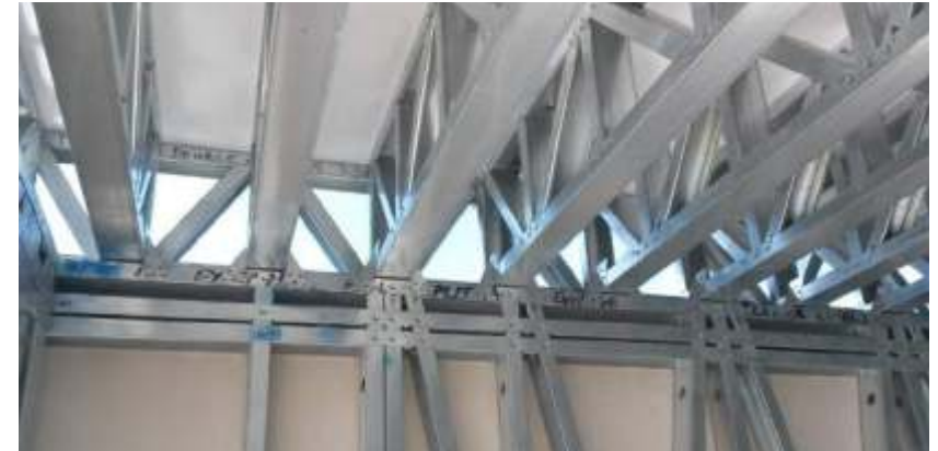
Light Steel Frame Joist Floor Anchored to Light Steel Frame Ring Beam
